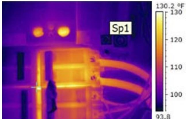
Photo set #3. Photo on left shows a 15 year old 150-amp power panel in a poultry house. The infrared photo at right shows the breaker is heated to about 130 degrees F, which means it is likely to fail or trip prematurely. The reason is that this breaker is feeding a second poultry house! Power should never be fed through one poultry house to another, but only from the farm main service.
